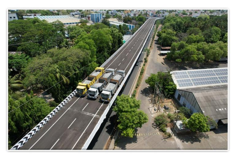
The load testing is used to check whether maximum deflection and percentage recovery are within permissible limits or not IRC SP:51
